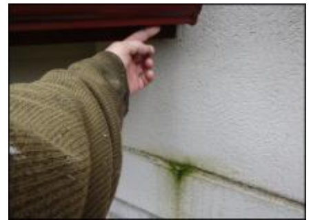
Leak at gutter end cap needs remediation (B4)
