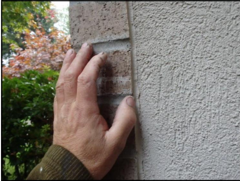
Sealant joint in good condition at EIFS to brick (E5-E7)
