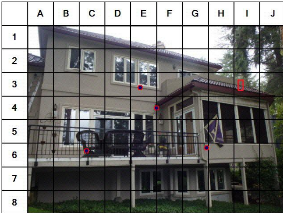
Exposed EPS at roof termination needs base coat and mesh application (F4)
