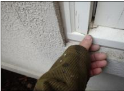
Window construction adequately sealed; typical
