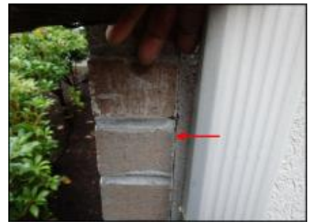
EIFS to brick needs sealant joint application (A1-B8)
