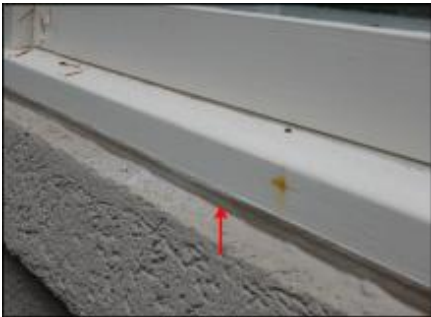
Sealant joint in good condition at window perimeter; typical
