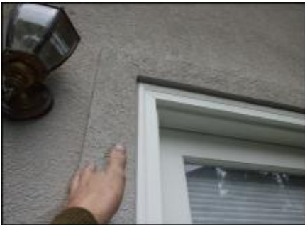
Sealant joint in good condition at door head and jambs; typical
