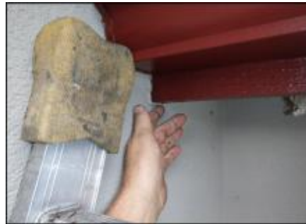
Sealant joint in good condition at fascia termination; typical
