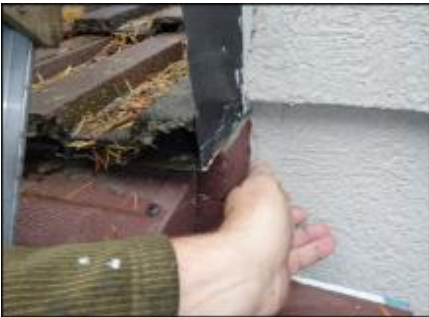
Sealant joint in good condition at roof termination; typical
