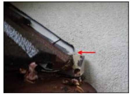
Sealant applied at secondary roof termination (E3)
