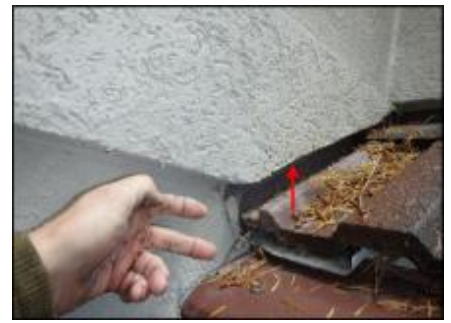
Exposed EPS at roof termination needs base coat and mesh application (F4)
