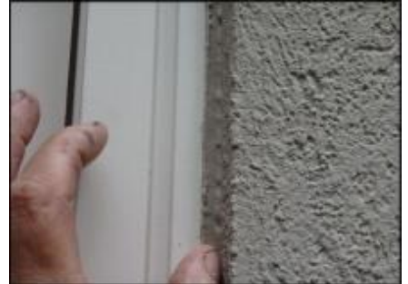
Sealant joint in good condition at window perimeter; typical
