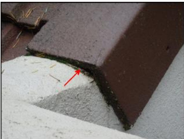
Recommend removing roof tile for elastomeric coating application (G2, H3)
