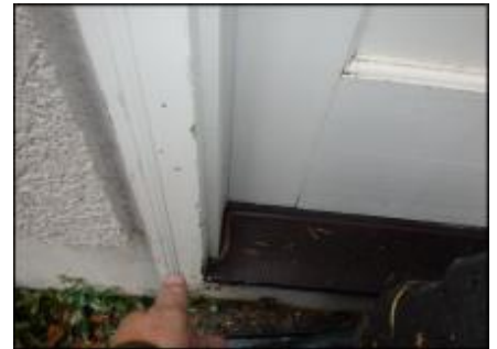
Sealant in good condition at door threshold (J7)
