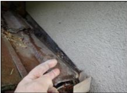
Sealant applied at secondary roof termination (H3)
