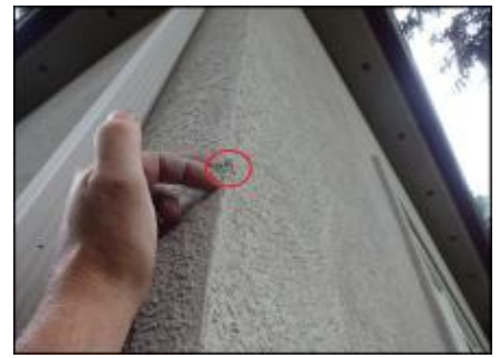
Area of impact damage needs remediation (C4)
