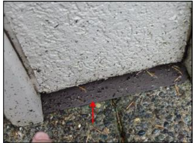
Flashing installed at base of system at garage
