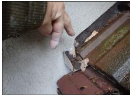
Sealant applied at secondary roof termination (G2)
