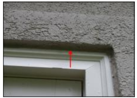
No drip flashing installed at window head; sealant joint installed; no remediation necessary; typical
