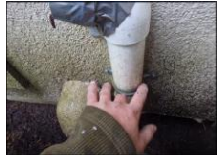
Utility fasteners need to be sealed (G6)
