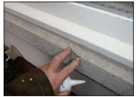
Area of impact damage needs remediation; typical of elevation
