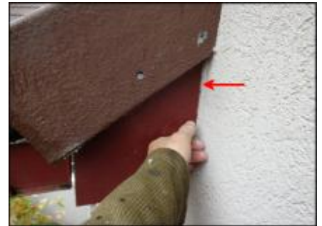
Sealant joint in good condition at fascia termination; typical
