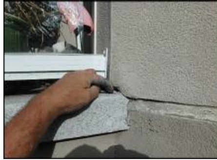
Deck termination need end dam flashing installation; typical
