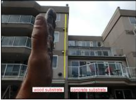
Wood substrate to concrete substrate needs expansion joint installation (H2-H6)
