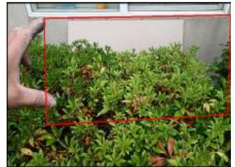
Approximate area of soft substrate needs to be removed and replaced (D7-E7)
