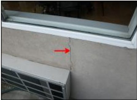
Cracks need to be gouged and slivered with EPS prior to base coat, mesh and finish coat application; typical
