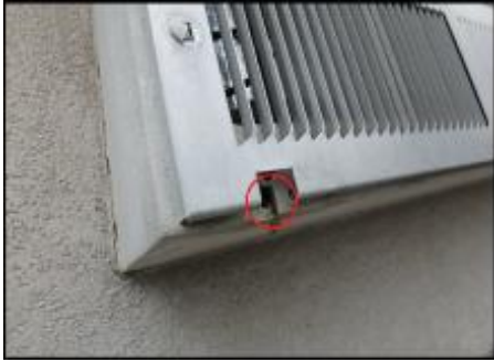
PTAC needs factory drip tubes installed to divert water away from system; typical
