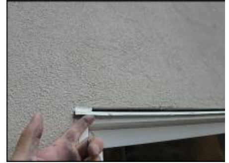
Head flashing with sealant end dams installed at remediated windows (C4-C7)
