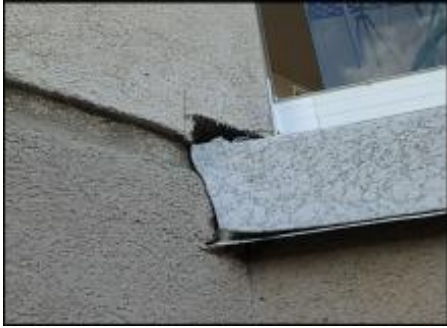
Recommend replacement of deck membrane due to installation defects and failure observed; typical
