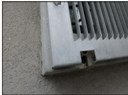
PTAC needs factory drip tubes installed to divert water away from system; typical
