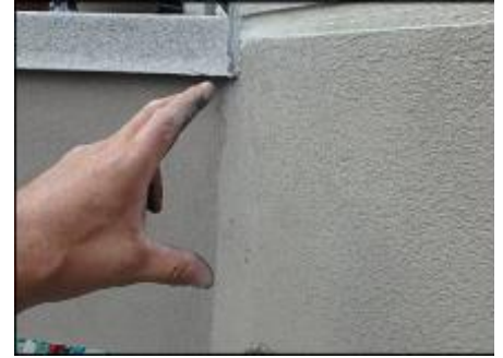
Inconclusive probing results below deck due to OSB substrate cut out to accommodate steel bracket installation; recommend random intrusive evaluation upon system remediation to determine framing condition; typical
