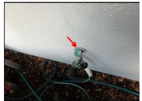
Penetration needs sealant joint application; typical
