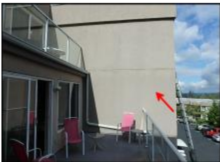
EIFS applied over concrete substrate at wall (B2-B5)
