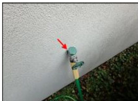
Penetration needs sealant joint application; typical
